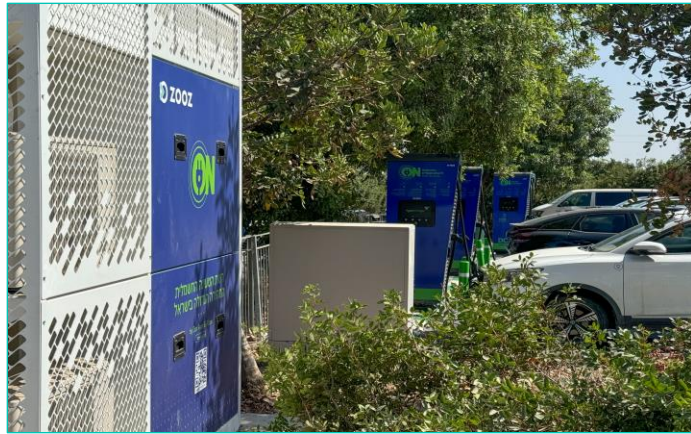
Several Installation WW
